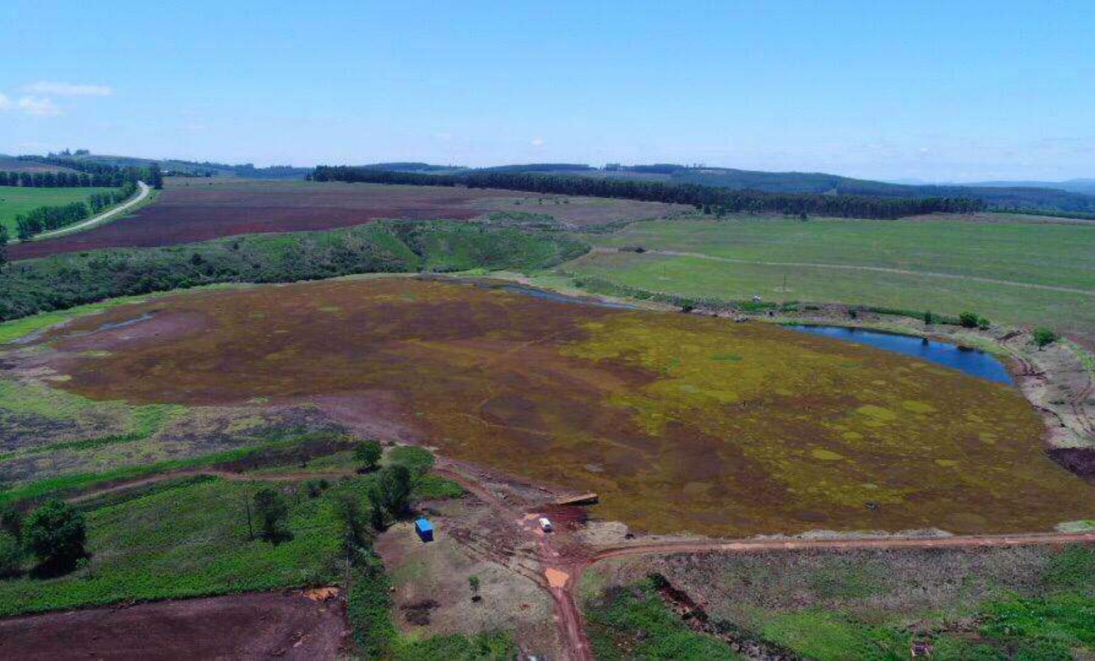
IXOPO DAM AT THE START OF THE PROJECT
