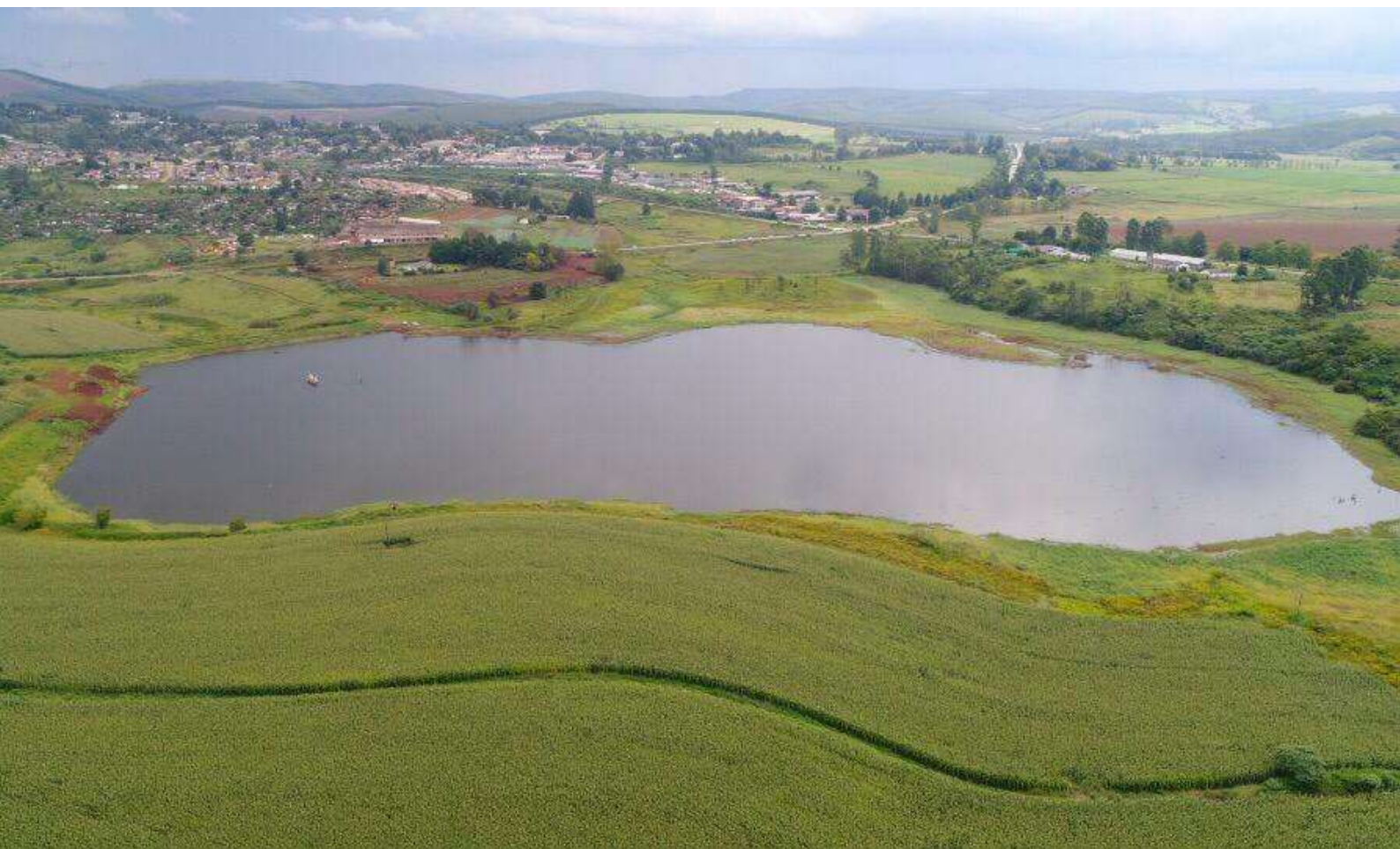
IXOPO DAM ON PROJECT COMPLETION
